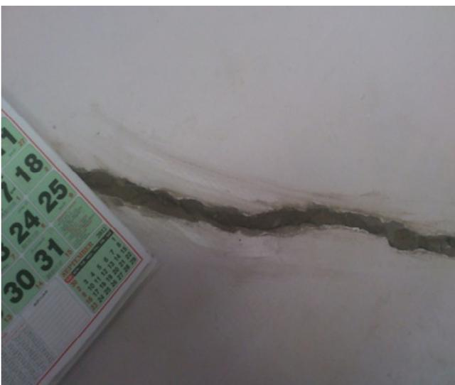
**CRACKS FOUND IN WALLS:** Cracks are found all over the buildings. The cracks are caused due to settlement of the structure due to the soil condition.
