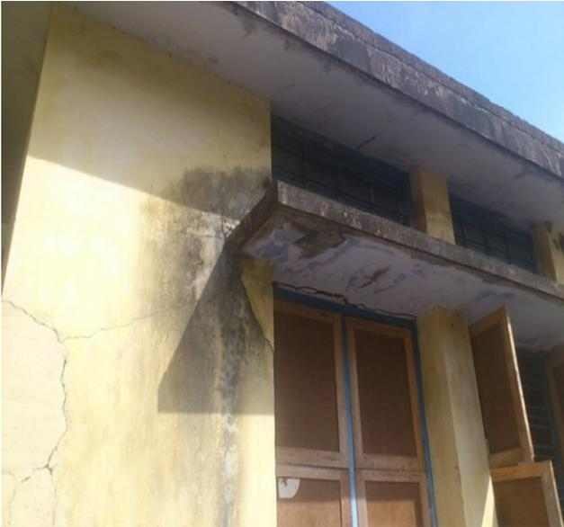
**WALLS & ROOF SPALLING:** Cracks and spalling of concrete found inside the wall. This is due to water penetration which causes reinforcement bars to get corroded. Due to corrosion the rods expand which leads to spalling in concrete surface.
