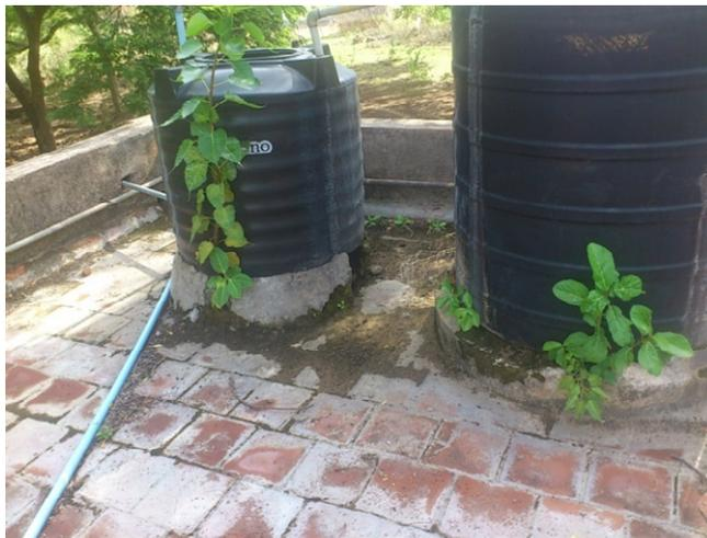
Further we find lot of vegetation grown over the flat roof which has damaged the roof and has allowed water to penetrate. The penetration of water dampness can be seen in MATERNITY WARD as shown in the picture.
